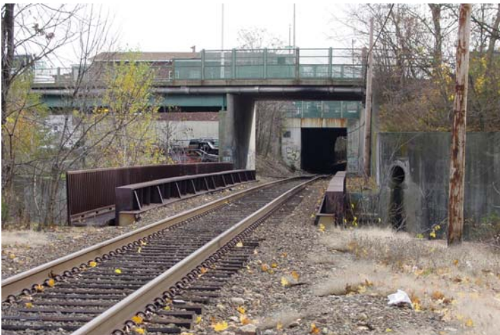
Undergrade & Overhead Bridges.
